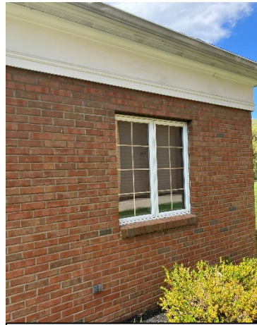
Brick Sill and Lintels
