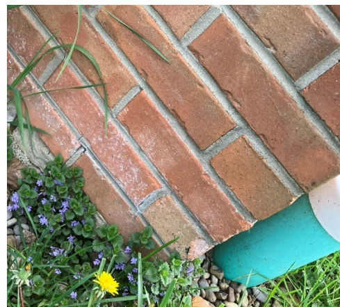
Mortar Deterioration and Spalling
